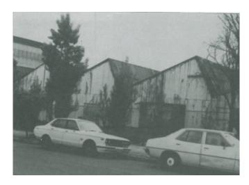
Figure 5:1984 photograph of the Shepherd Street (west) facade of the factory showing the earlier corrugated iron cladding that was identified as being of heritage interest
