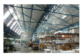
Figure 7: Interior of the factory building, looking west towards Shepherd Street, showing the saw tooth roof structure
