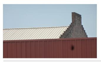
Figure 11: Brick gable to the party wall at the southern end of the post 1943 eastern addition to the factory at 61-65 Shepherd Street
